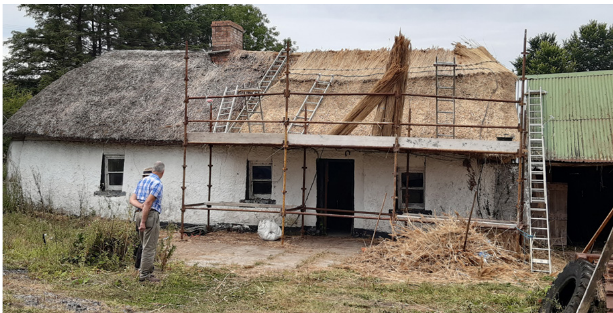
Rethatching Clonaboy 2022 funded by the Built Heritage Investment Scheme
