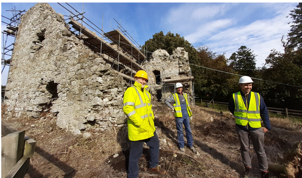
Site meeting, during conservation works at the 'Leper Hospital' in Kilbixy
